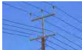
High voltage and low voltage on same pole
